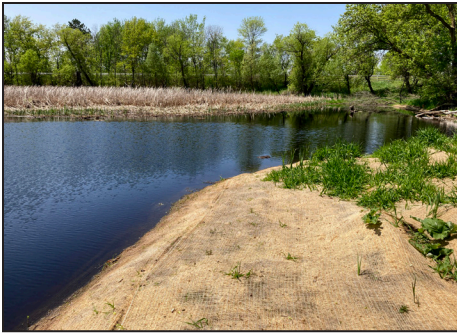
Left: Erosion control measures and native plants were installed after 1,480 cubic yards of sediment was removed from this half-acre wetland bordering Moody Lake in February. The material was spread on neighboring cropland. This wetland restoration will keep an estimated 47 pounds of phosphorus out of Moody Lake each year. Moody Lake drains to Bone Lake. Middle: Doug Tovos of the Comfort Lake-Forest Lake Watershed District Board of Managers, left, and CLFLWD Administrator Mike Kinney discussed the Clean Water Fund-backed project. Tovos donated easements granting the CLFLWD 25 years' access to the project area and four years' temporary access to another 0.22 acre. Right: A now-empty dairy barn stands next to the wetland. VIDEO
