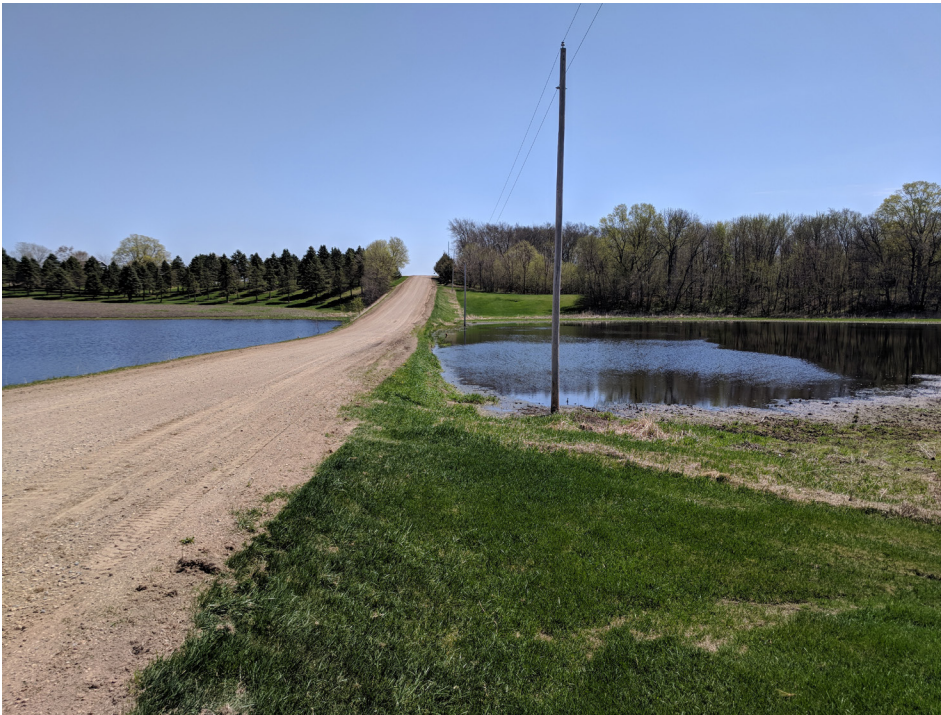
The Le Sueur County Highway Department will replace a culvert under County Road 138 to provide additional protection for the road embankment and right-of-way. The culvert work is one component of the project to restore a wetland on Jeff and Christy Gibbs' farm.
